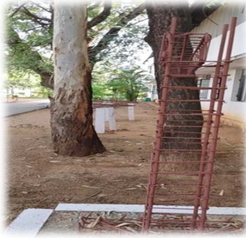
Typical Column Reinforcement with lateral ties
