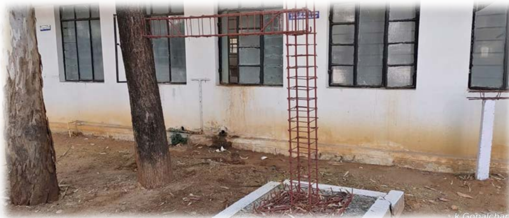
Beam Column and Footing Reinforcement
