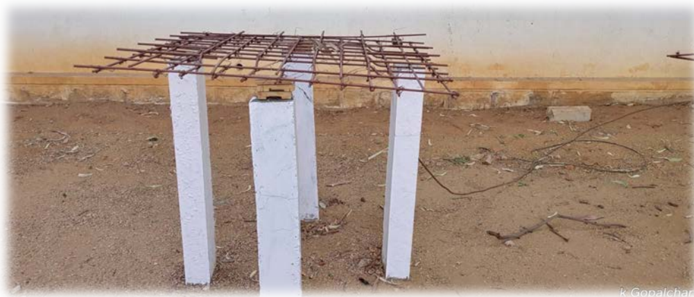
Two way slab reinforcement
